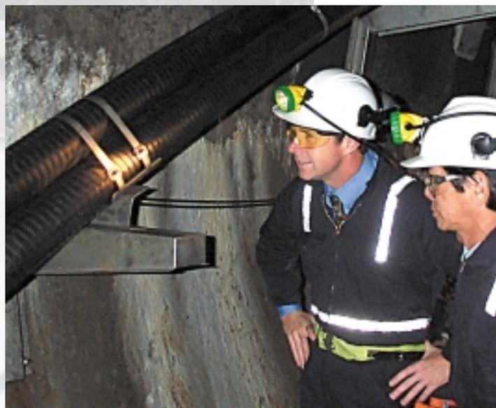
Underground cable in New Zealand is secured with fireproof BAND-IT stainless steel clamps
