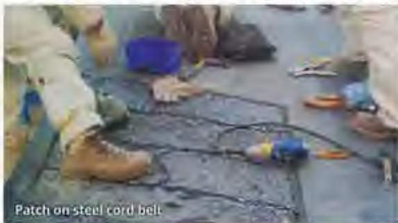
Patch on steel cord belt
