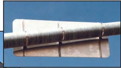
Mast Arm Sign Installation
