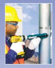
Is installation time critical? Field tests show that Ultra-Lok clamps can be applied four times faster than conventional band clamps.
