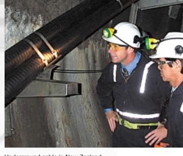
Underground cable in New Zealand is secured with fireproof BAND-IT stainless steel clamps
