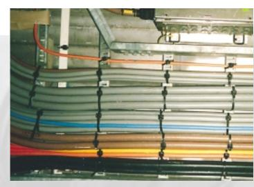
Reusable BAND-IT Ties are coated with Nylon 11 for superior corrosion resistance in this marine cable bundling application. The coating also protects cable from damage or interference due to direct contact with stainless steel.
